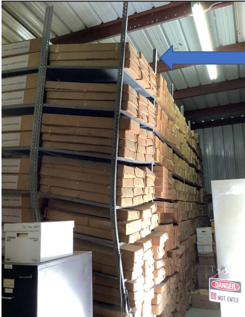
Earthquake bracing is not secured
